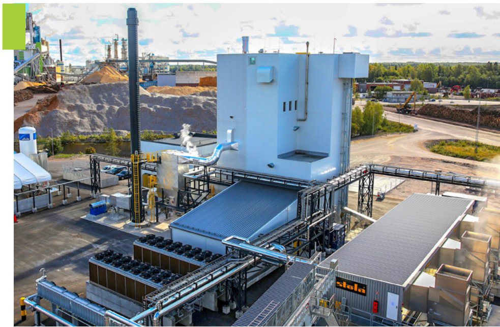
Second-generation fast biomass pyrolysis plant (Fast Pyrolysis Bio-Oil or FPBO) produces biofuel at Gävle, Sweden
