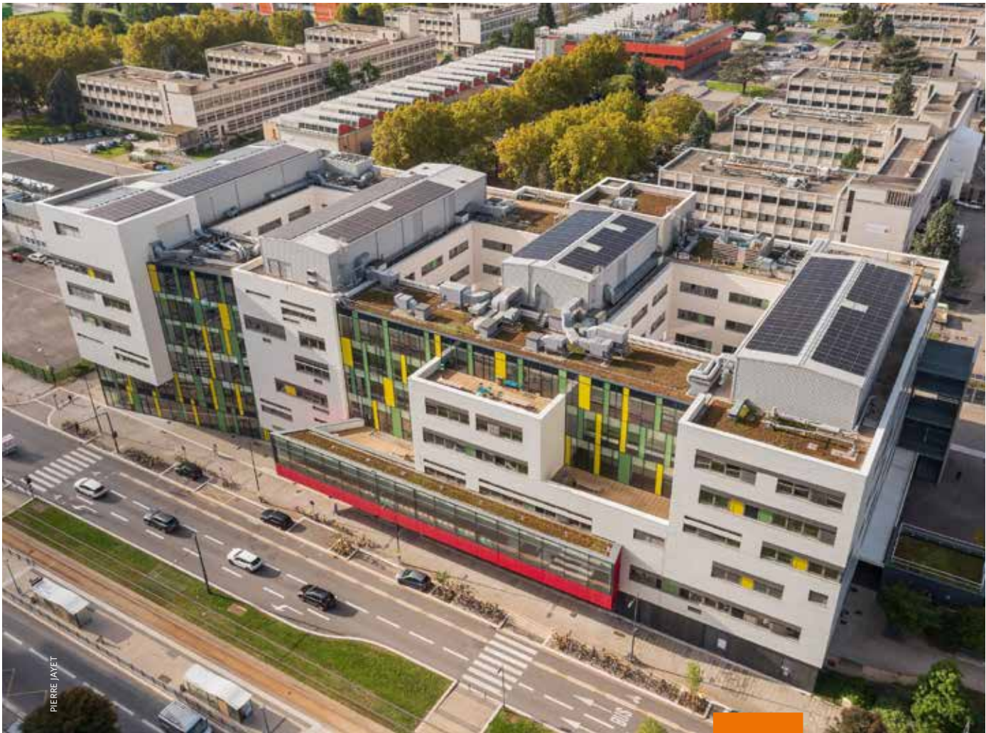
In March 2023, a self-consumption roof-mounted power plant went on stream on the University of Grenoble campus. It is installed on the roof of the GreEn-ER building, that accommodates an engineering school and a research laboratory. This 195-kW power plant will cover 10–15% of the building’s electricity demand (23 000 m² and 2 000 occupants).
