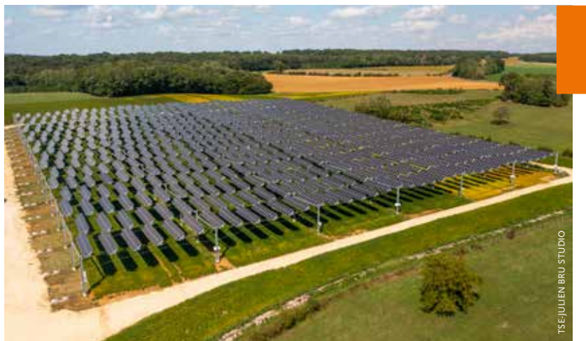
In 2022, TSE, the independent solar energy producer, inaugurated its first agrivoltaic demonstrator on field crops at Amance, in the Haute-Saône. The project is integrated at the heart of an 850-hectare farm. The canopy covers 3 hectares of crops including: soya, wheat, forage rye, winter barley and rapeseed with 2.4 MW of generating capacity.
